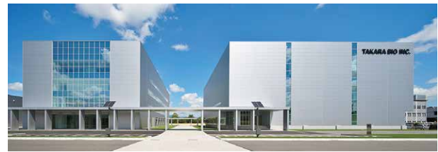
Main Research Building
